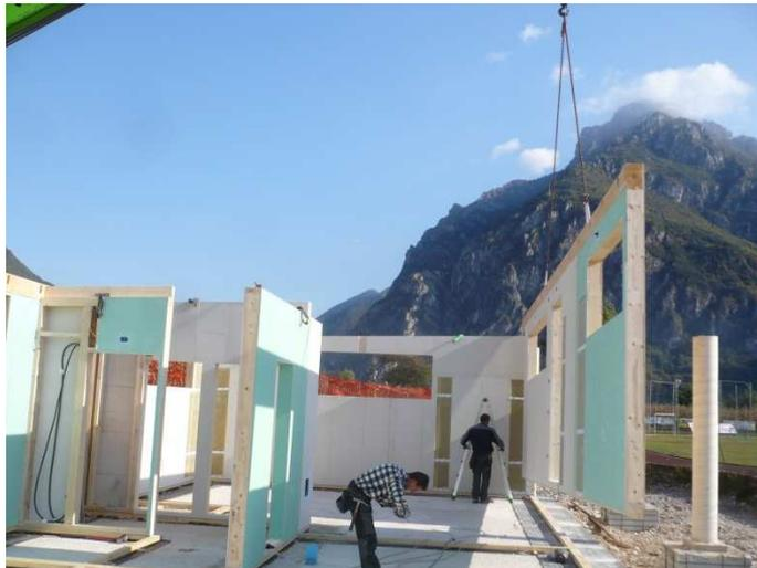
**Figure 1.3:** *Prefabricated wall placing in situ*
