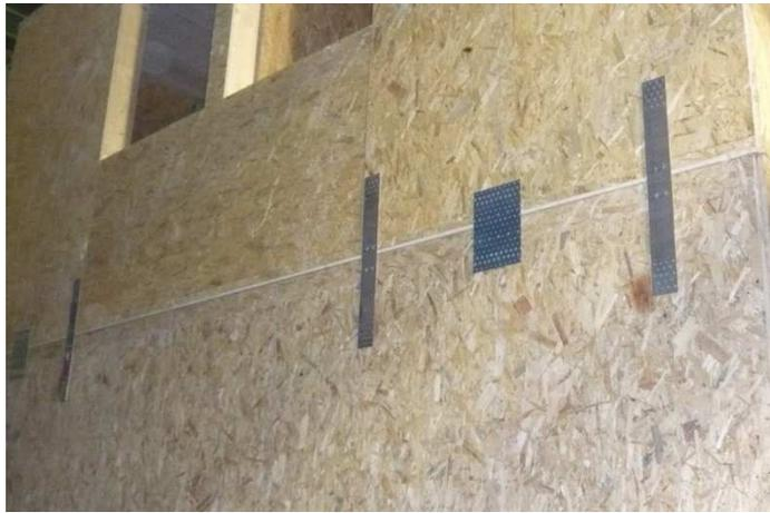
**Figure 2.10:** *Nailed steel plates for upper wall connection*
