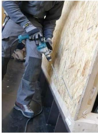
**Figure 6.5:** *Inclined screws connection*
