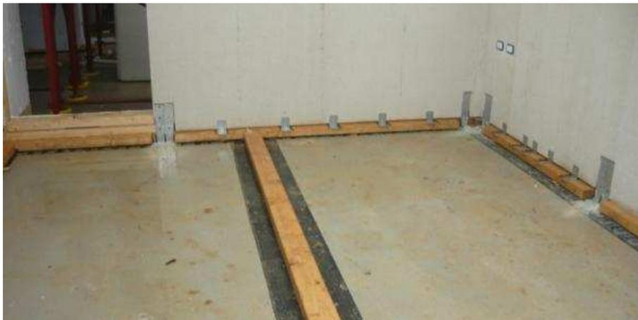
**Figure 2.5:** *Hold-down and Angle brackets positioning*
