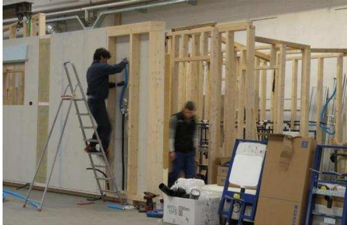
**Figure 1.2:** *Timber frame wall assembling in the factory*
