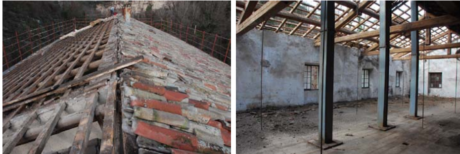
Figure 4.12 _ roof covering substitution
