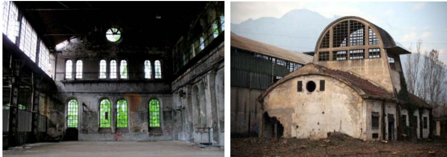
Figure 1.5 _ Interior (left) and exterior (right) of two Italian forsaken industrial buildings
