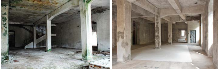
Figure 4.7_ ground floor spaces before and after cleaning
