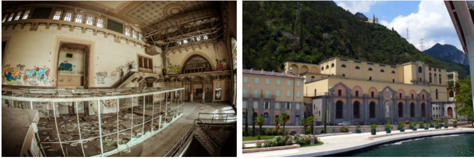
Figure 1.3 _ Interior (left) and exterior (right) of two Italian hydroelectric central buildings of the beginning of XX century.
