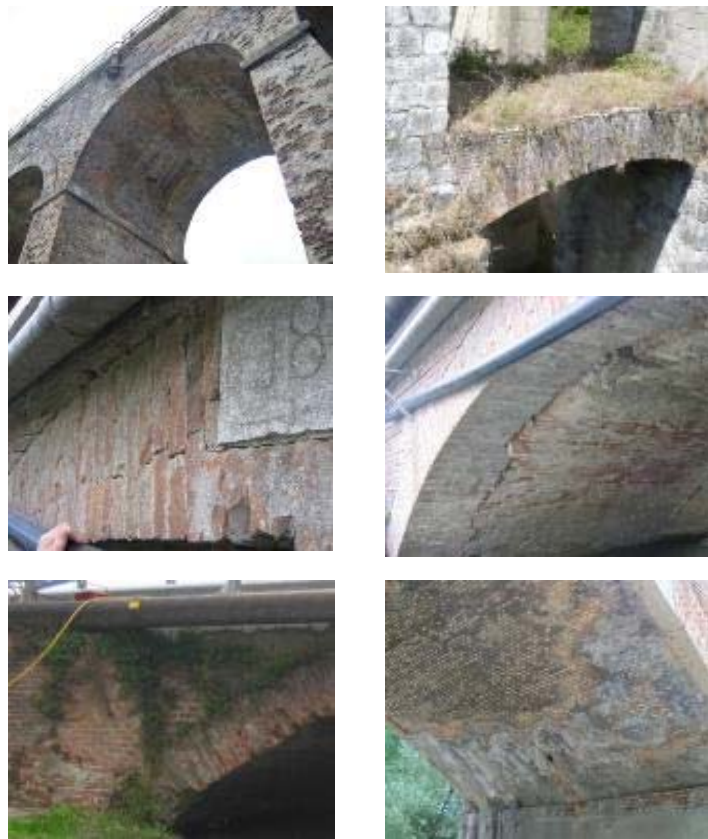
Fig. 2.8 Typical defects of masonry arch bridges. Loss of bricks, longitudinal cracking in barrel vault; opening of arch joints, salt efflorescence in bricks; penetration by vegetation.
