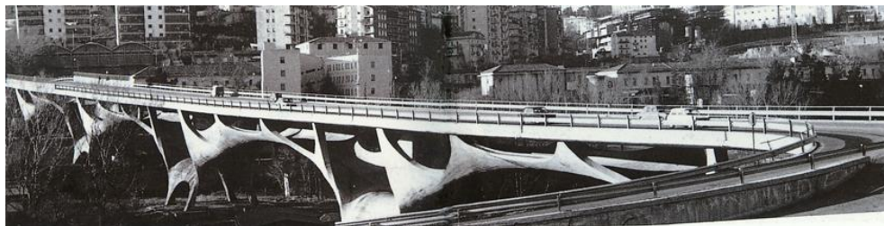
Fig. 8 Basento Bridge - S. Musmeci, 1969, Potenza (Italy)
