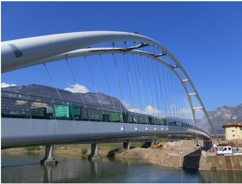
Figure 4.4: San Michele Footbridge.
