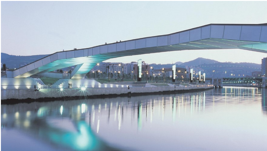
Figure 4.11: The Bilbao footbridge.
