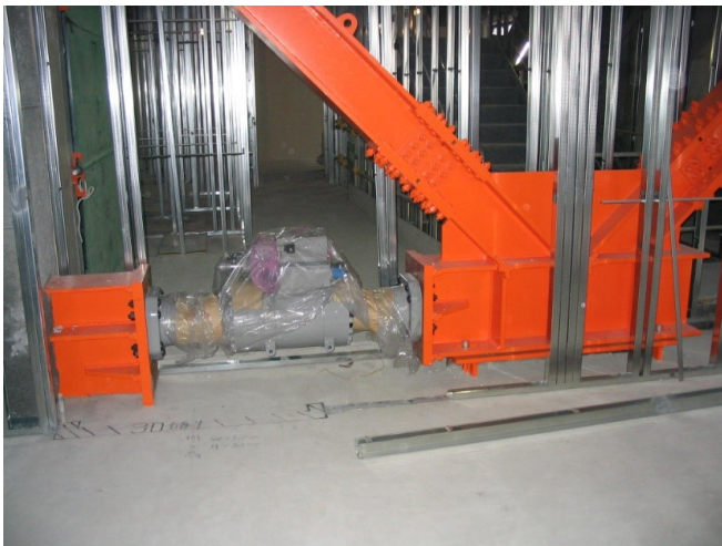
Figure 4.10: Kajima Shinozuka Building - semi-active hydraulic damper.
