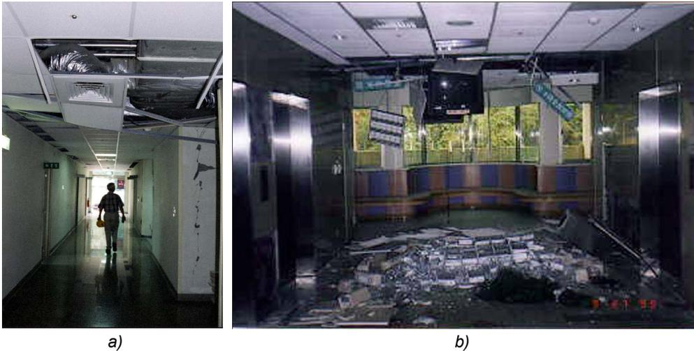
Fig. 2.3 Damage to the non-structural components and contents of the Veteran Hospital (a) and Shiu-Tuan Hospital (b) (from Soong & Yao, 2000).
