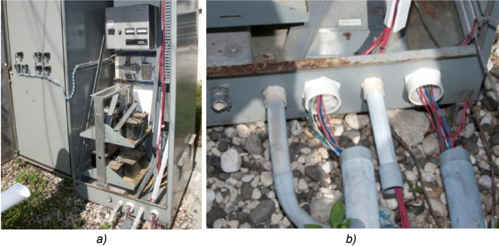
Fig. 2.4 a) General purpose cabinet, unanchored, at General Hospital of Haiti. b) Control wiring conduit damage after 2010 Haitian quake (PGA=0.21g). (From Goodno et al., 2011).
