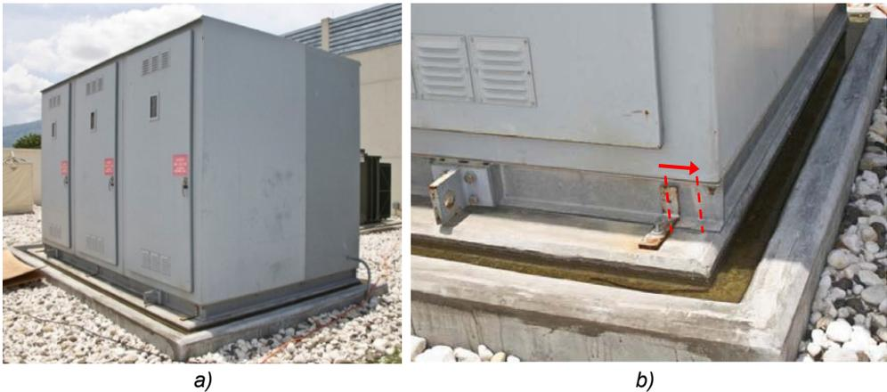
Fig. 2.5 a) Metal-enclosed load interrupter switchgear (MELIS) equipment at the U.S. Embassy. b) Displacement due to the 2010 Haitian quake (PGA=0.16g). (From Goodno et al., 2011).
