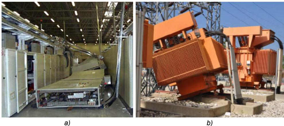
Fig. 2.6 a) Electrical cabinets overturned by 1999 Izmit earthquake –magnitude 7.4- Turkey (photos of NISEE Izmit Collection). b) Rail mounted transformer slipped off rails by 2010 Haiti earthquake –magnitude 7- Port-au-Prince (photos of Eduardo Fierro, BFP Engineers). (From FEMA E-74, Jan. 2011).
