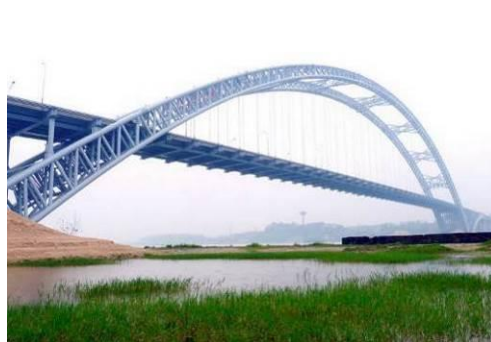
e) Maocaojie Bridge, Hunan, China
