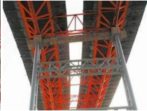
b) Bottom view of the truss girder
