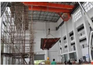
j) Lifting girder
