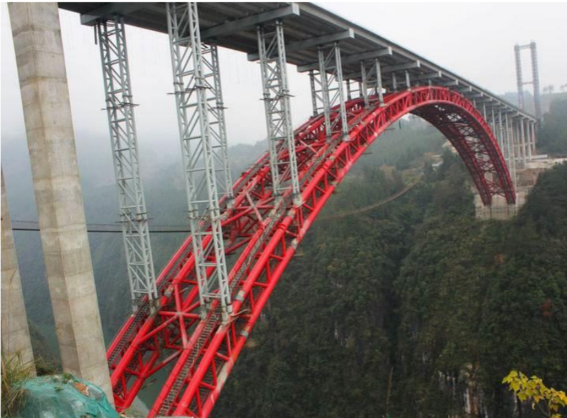
Fig. 11 CFST built-up columns used for pillar (Mengdonghe River Bridge, Hunan, China, completed in 2013)
