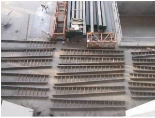
d) Segment of column
