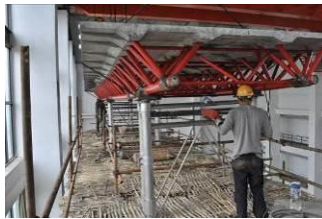
k) Welding girder and columns
