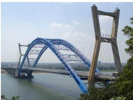
d) Liancheng Bridge, Hunan, China
