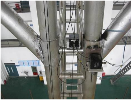
a) Accelerometers on the column
