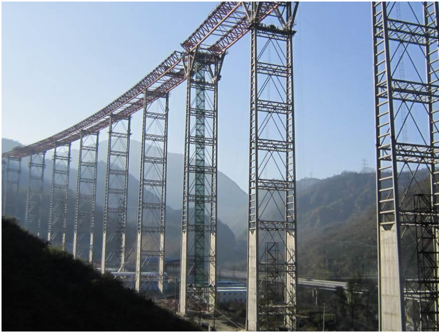
Fig. 12 CFST built-up columns used for continuous beam bridge (Ganhaizi Bridge, Sichuan, China, completed in 2012)
