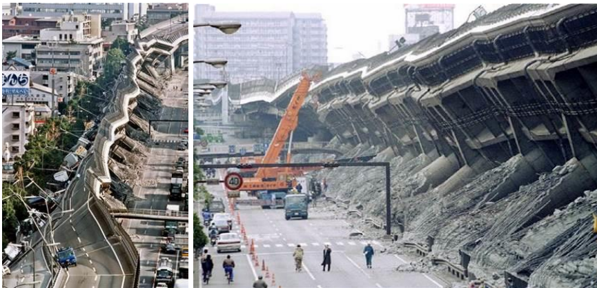
Fig. 15 Flexural failure of the whole bridge, Hanshin Expressway, Kobe Earthquake, Japan, 1995
