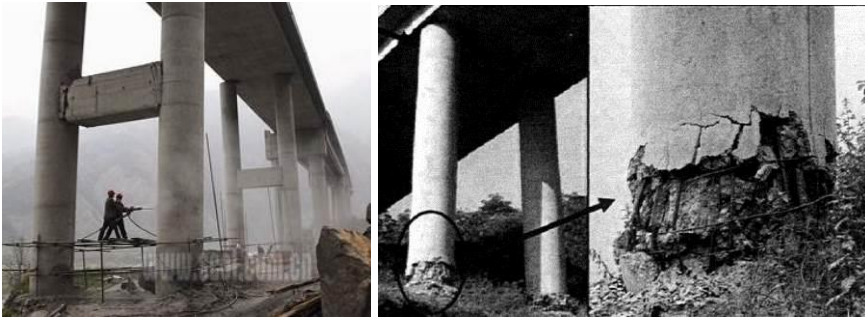
Fig. 16 Shear failure of the tie beam and flexural failure at the base of column, Baihua Bridge, Wenchuan Earthquake, China, 2008
