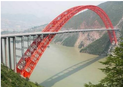
b) Wushan Bridge, Chongqing, China
