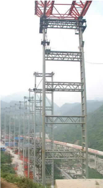
c) Transverse view of the pier
