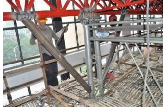
l) Welding slant supports
