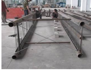
e) Positioning of column
