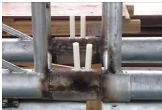
h) Grouting joint of column
