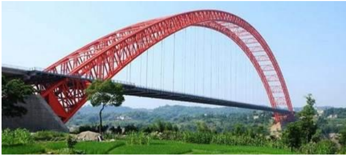
a) Bosideng Bridge, Sichuan, China
