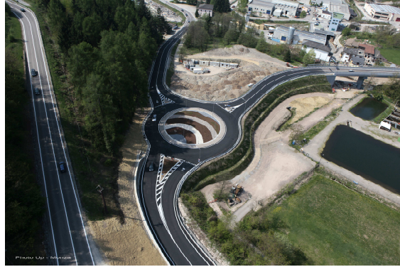
Figure 7.1: Aerial picture of the Torchio roundabout, embankment, and bridge abutment ( http://www.provincia.tn.it/ ).
