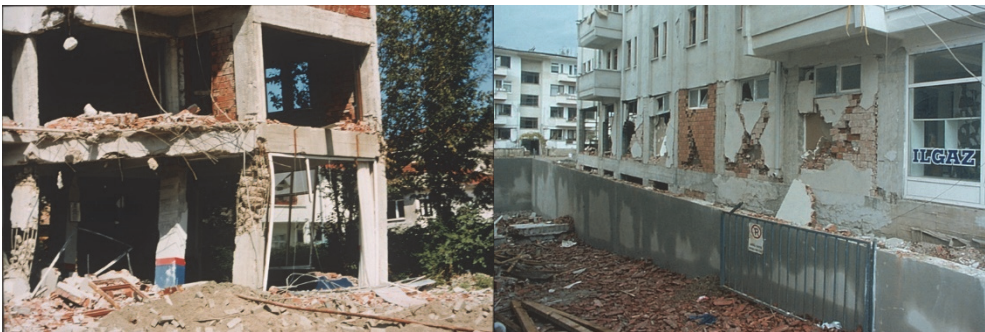
Fig. 1.3 Damage and collapse of infill walls in 1999 Turkey earthquakes. Left: August 17 Izmit (Kocaeli) earthquake. Image credit: NOAA National Geophysical Data Center. (NOAA 2007) Right: November 12 Düzce earthquake. Image credit: NOAA/NGDC, Roger Bilham, University of Colorado, Dept. of Geological Sciences.
