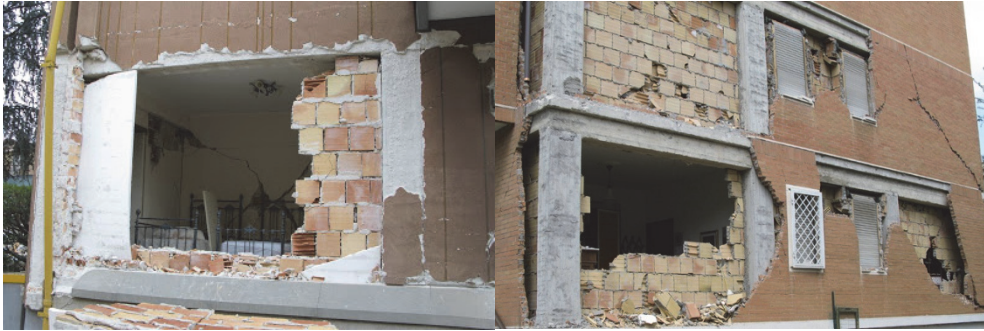
Fig. 1.5 Damage to clay blocks infill walls after 2009 L'Aquila earthquake, Italy. Left: Image from (Scott 2009). Right: Image from (Miyamoto 2013).
