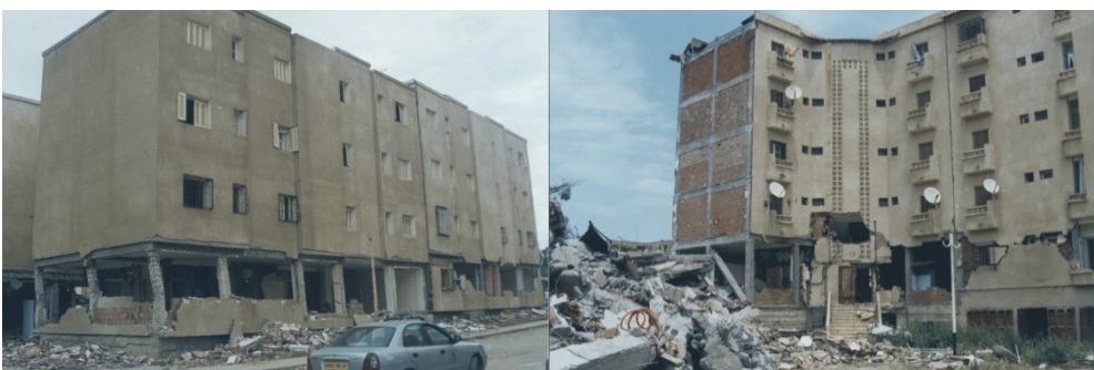
Fig. 1.4 Damage to infill walls after 2003 Boumerdes and Algiers (Algeria). Image credit: NOAA/NGDC, Djillali Benour. University of Bab Ezzour, Algeria.
