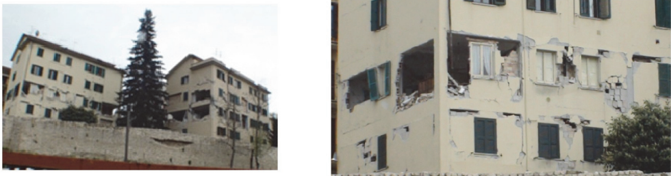
Fig. 3.2 Collapsed infill walls located at upper-storeys as a result of IP/OOP interaction in L'Aquila 2009 earthquake. Image from Günay and Mosalam (2010b).
