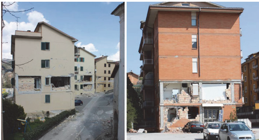
Fig. 2.1 Out-of-plane collapses of masonry infill walls. Image from (Braga et al. 2010). Note that the most damaged panels are typically localized at the lower stories, albeit not necessarily at the first storey.
