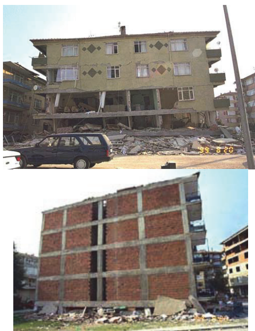
Fig. 3.3 Formation of soft storeys following URM infill wall collapses in 1999 İzmit (Kocaeli) earthquake, Turkey. Image taken from Sezen et. al (2000).
