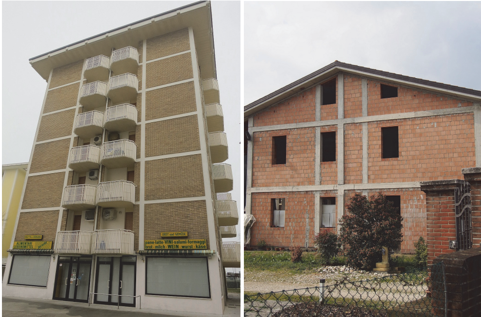
Fig. 1.1 Examples of typical usage of URM infill walls in residential RC frame structures. Showing a six storey condo in Bibione (VE), and low-rise family house under construction in Cusignana (TV).
