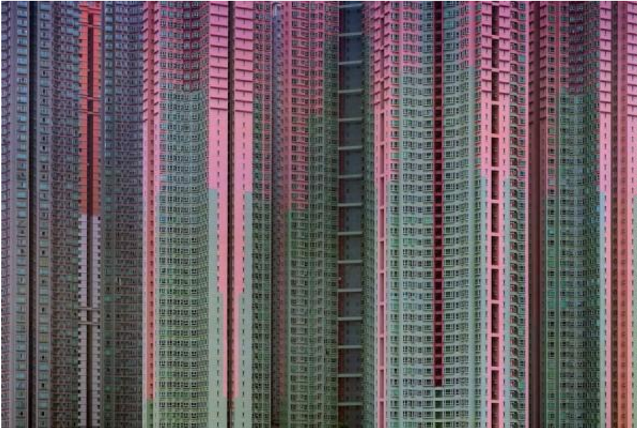
Fig. 1.21: Typological weaknesses: unprepared to deal with relentless design outputs of large numbers: Housing towers, Shenzhen, China
