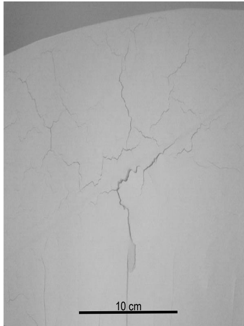
Figure IV – 2. Cracked green material because of an incorrect drying process
