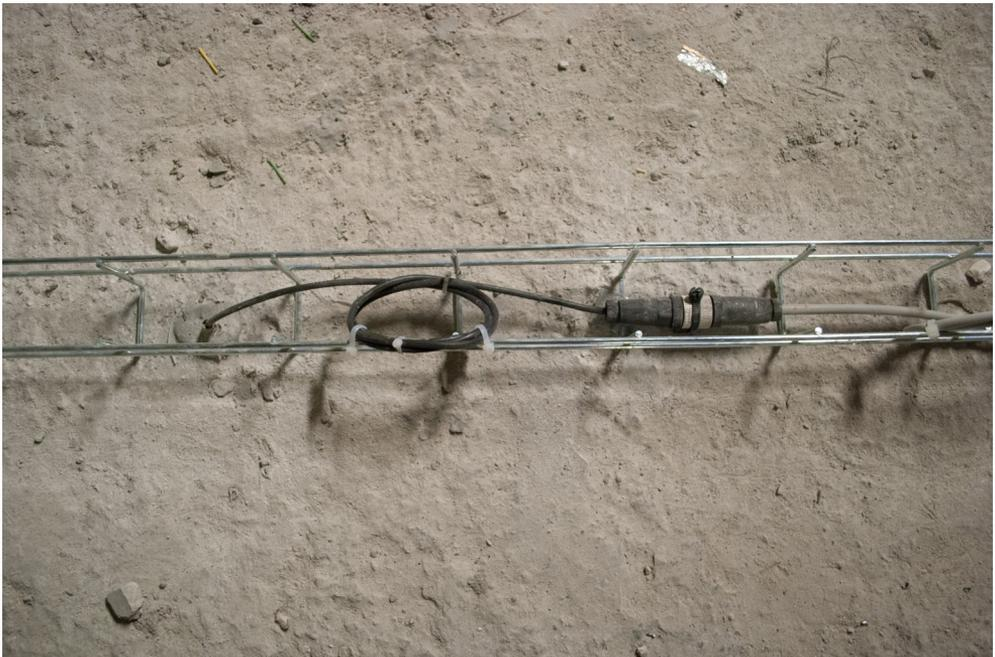
Figure 6.11. A RTD installed on the bottom slab of southbound southernmost girder of Colle Isarco Viaduct.
