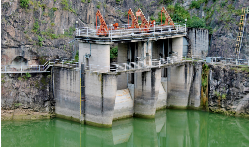
Figure 7.1: Sluice gates of the Stramentizzo dam (Italy).
