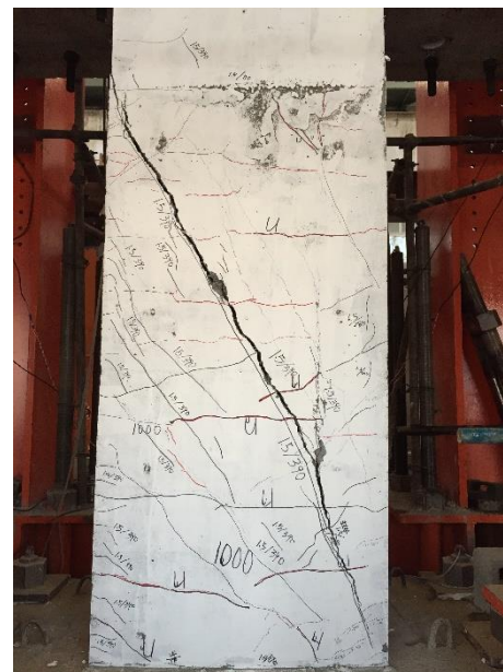
(b) Crack distribution in back view
