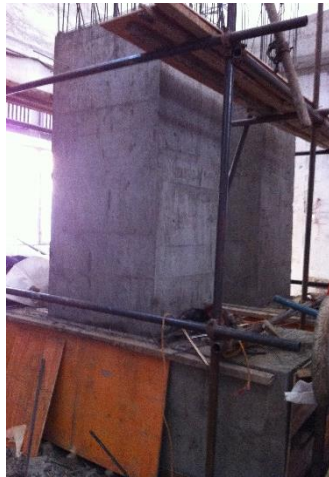
(a) Base and the pier part below the clapboard
