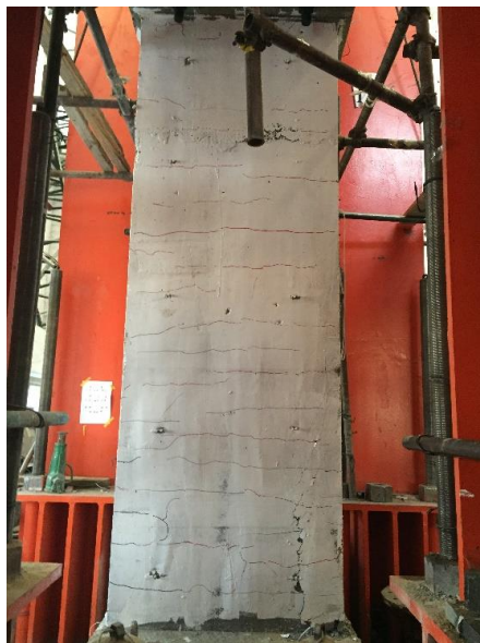
(a) Crack distribution in the right elevation
