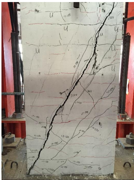
(a) Crack distribution in front view
