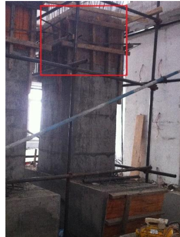
(b) Clapboard and the pier part above
