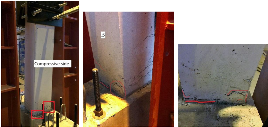
Fig. 4-7 Photos of the specimen after testing-View of compressive side
