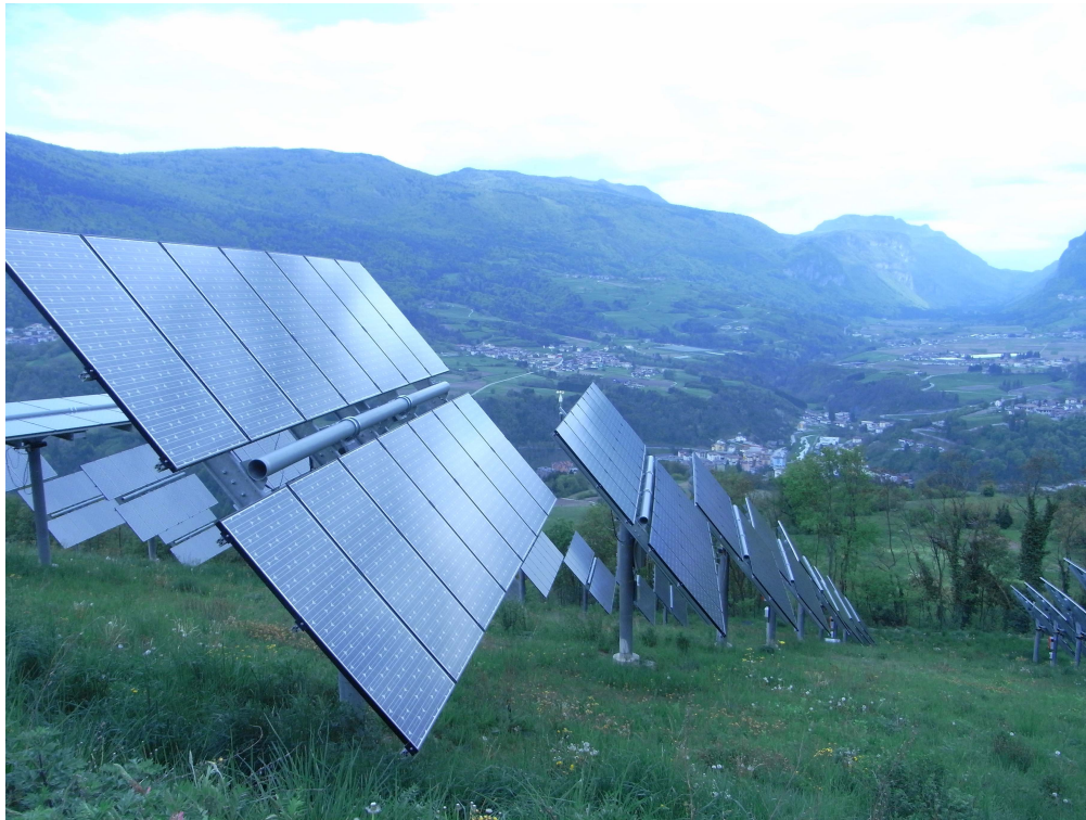
Figure 2 Photovoltaic installation in Storo
