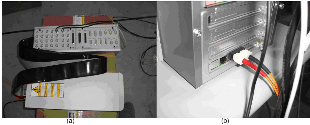
Fig. 9.8: (a) PPC 1103 unit and its connector panel; (b) detail of optical fiber connection to PC
