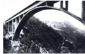
Passaro Bridge Costa river, Italy 1961, 100 m span
