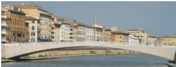
3. 48 Mezzo Bridge, Arno River, Pisa, 1948-50, 72 m span, G. Krall
