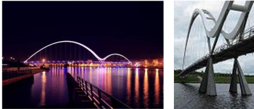
2. 23 Infinity Bridge, Stockton (UK), 2009, 120 m span, 32 m height, Expedition Engineering, Spence Associates.
