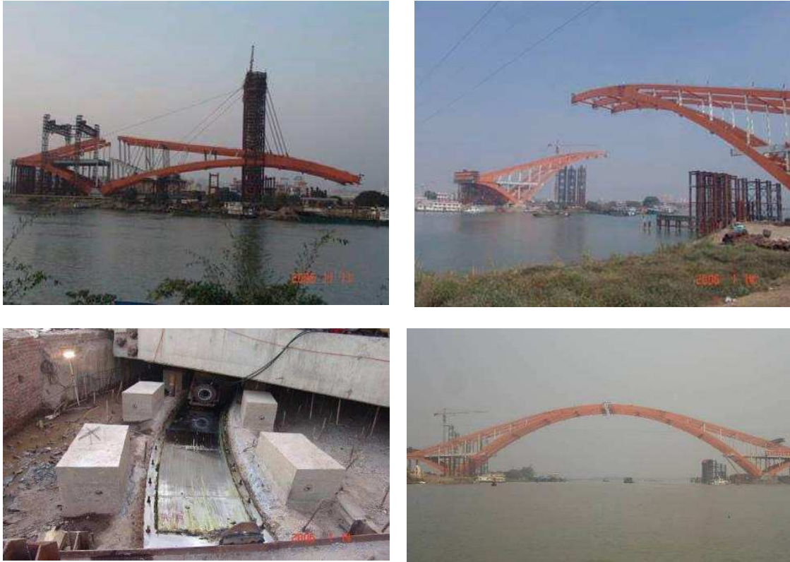
4. 61 Dong ping Bridge, China, 2006, 300 m span, construction phases
