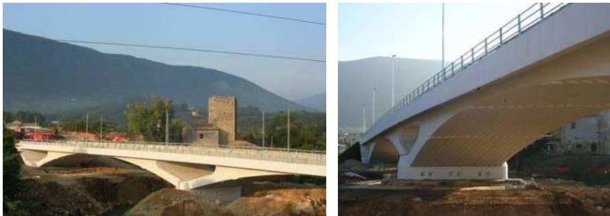
4. 70 Sgurgula Bridge, Rome, 2005, 56 m span, E. Siviero
