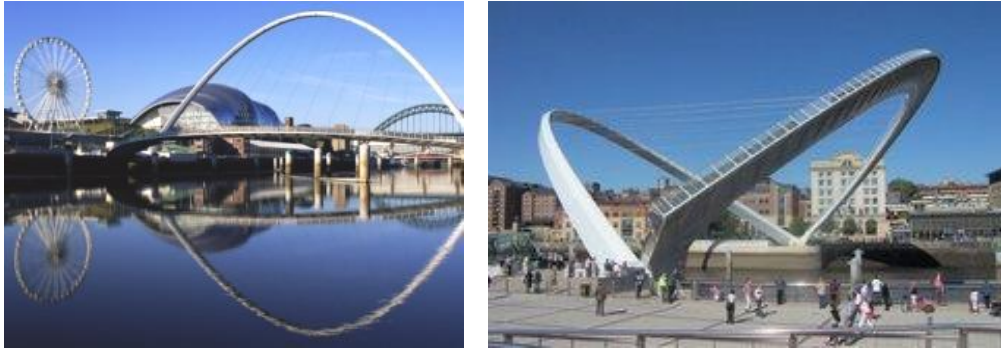
2. 26 Gateshead Millennium Bridge, Gateshead, UK, 2001, 105 m span, Wilkinson Eyre
