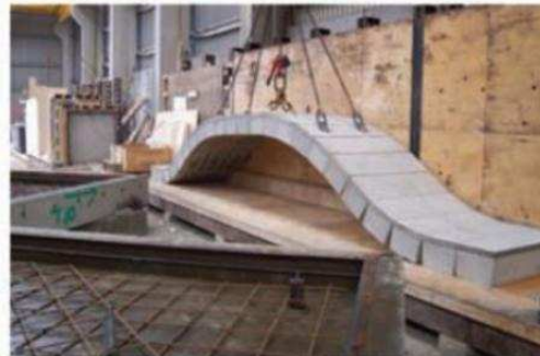
b. Arch Unit during Lifting
