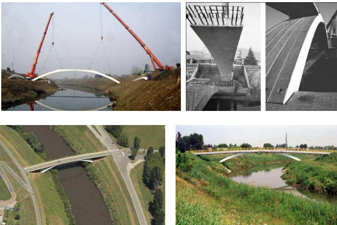
4. 68 Bicycle and Pedestrian Bridge at Ponte San Nicolò, Padua, 1998, E. Siviero
