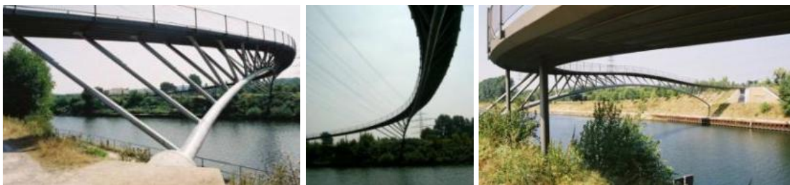
2. 27 Ripshorst Footbridge, Oberhausen, Germany, 1997, 78 m span, J. Schlaich, Bergemann and Partner
