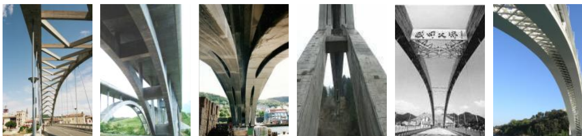
3. 31 Examples of different connection typologies between the ribs
