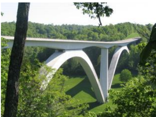
2. 7 Natchez Trace Parkway Bridge, Tennessee, USA, 1994, 177,4 m span, 44,2 m height, Florida-based Figg Engineering Group
