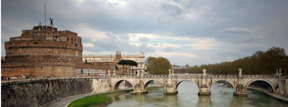
1. 16 Sant'Angelo Bridge, five spans of 18 m, 135 m total length, completed in 134 B.D., Rome
