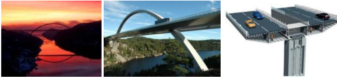
2. 15 Svinesund Bridge, connection between Sweden and Norway, 2005, 247 m span, 30 m rise, R. Schubart, B. Berger
