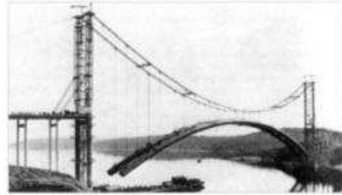
4. 28 Cable-stayed cantilever construction as in suspension bridge and Askerofjord Bridge, Sweden, 278 m span, 1961.
