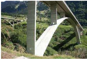
Nanin Bridge Mesocco, Grisons, Switzerland 1967, 112 m span
