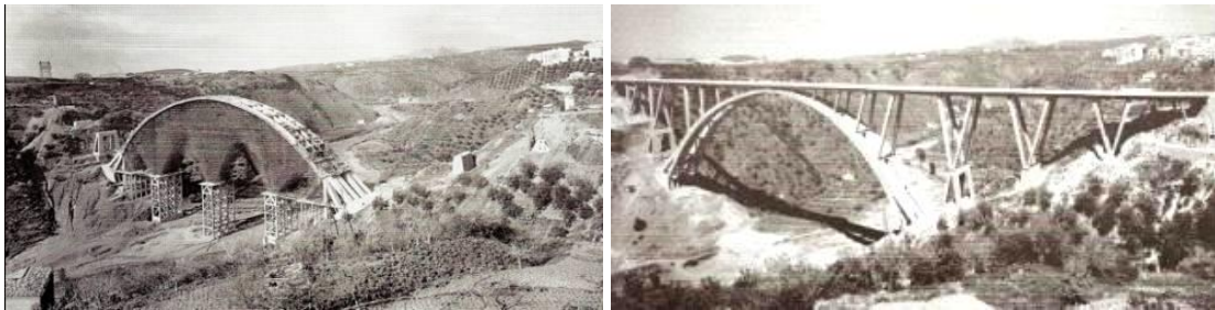
3. 51 Fiumarella Viaduct, Catanzaro, 1962, 231 m span, R. Morandi
