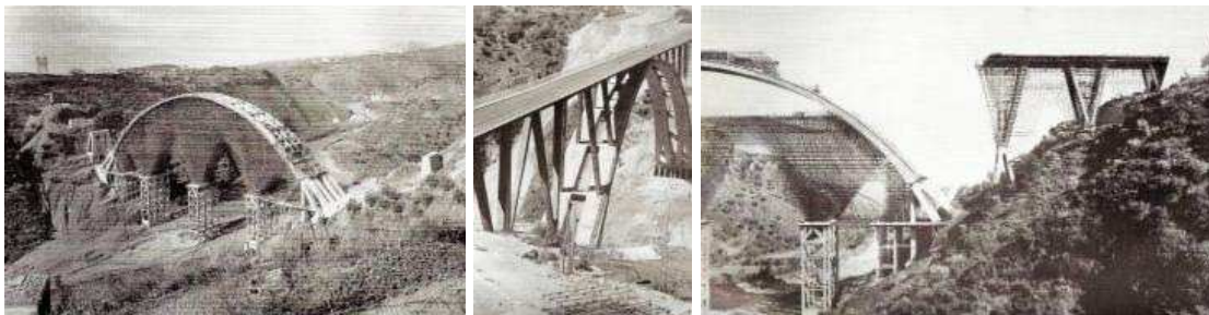
4. 5 Fiumarella pictures: construction phase and state of art Fiumarella Viaduct, Catanzaro, Italy, 231 m span, 1962, R. Morandi
