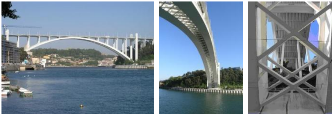
2. 2 Arrabida Bridge, Porto, Portugal, 1963, 270 m span, 52 m rise, E. Cardoso
