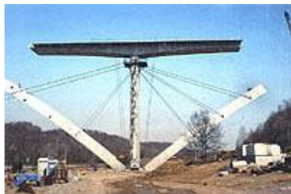
2. 7 Natchez Trace Parkway Bridge, Tennessee, USA, 1994, 177,4 m span, 44,2 m height, Florida-based Figg Engineering Group
