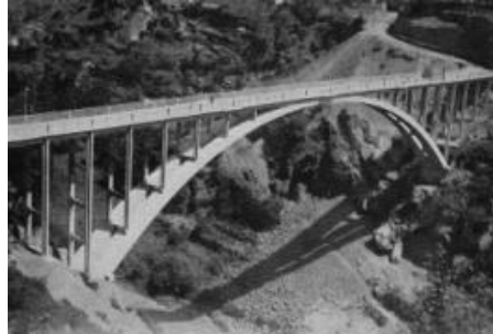
3. 44 Biedano Bridge, Viterbo, 1937, 91 m span, G. Krall
