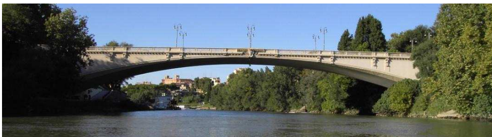
1. 52/a Risorgimento Bridge (picture and project), Rome, Italy, 1911, 100 m span, F. Hennebique
