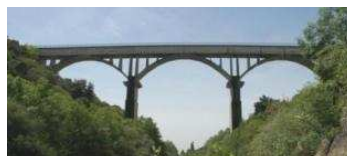
Alagon River Aqueduct 1966, 4 x 60 m span
