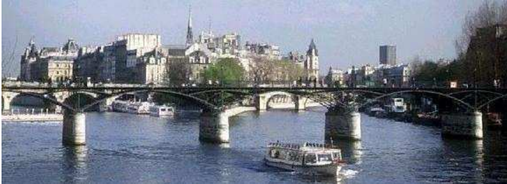
1. 35 The Pont des Arts, Paris, France, 1803, 18.5 m span
