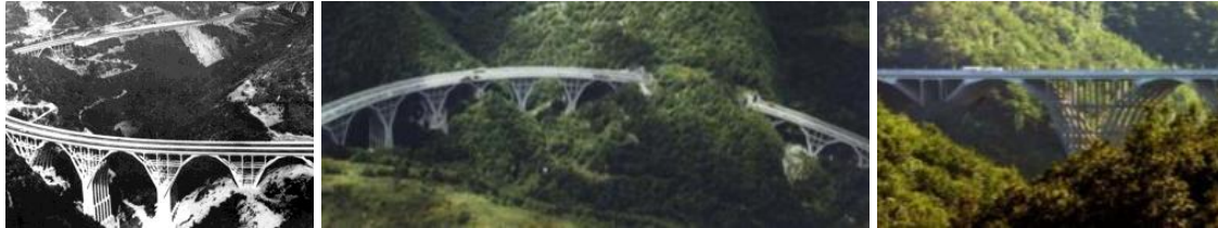
2. 13 Poggettone and Pecora Vecchia Viaducts, Sole Motorway, Italy, 1960, total length 455 m, 8 polygonal arches, A. Carè, G. Giannelli
