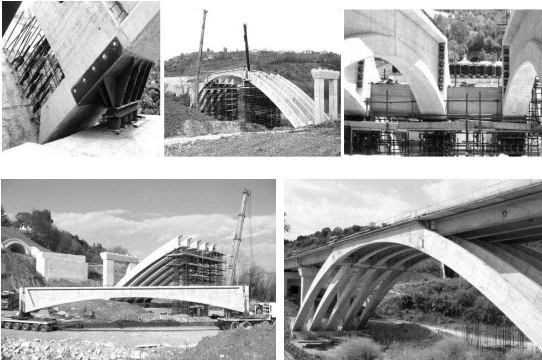
4. 71 Mazzocco Bridge, Pescara, Italy, 2007, 70 m span, M. P. Petrangeli
