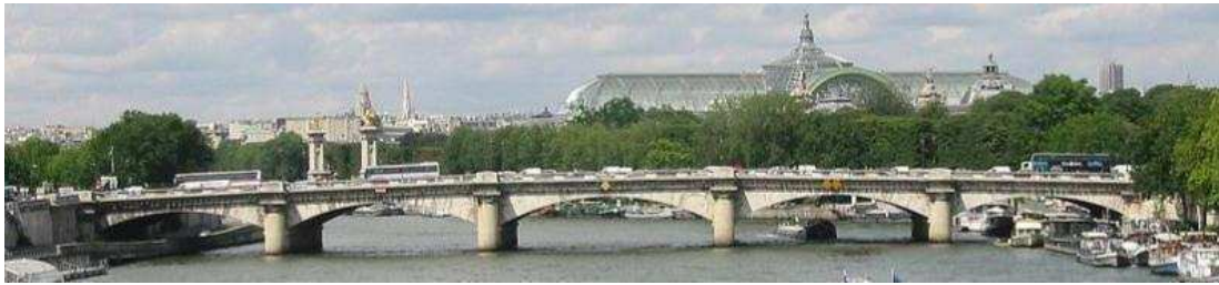
1. 33 Pont De La Concorde, Paris, France, 1791, 25 m - 28 m - 31 m - 28 m - 25 m span, J. R. Perronet
