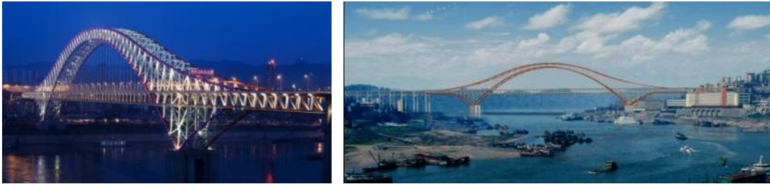
2. 22 Chaotianmen Bridge, 552 m span, 2008, Chongqing, China
