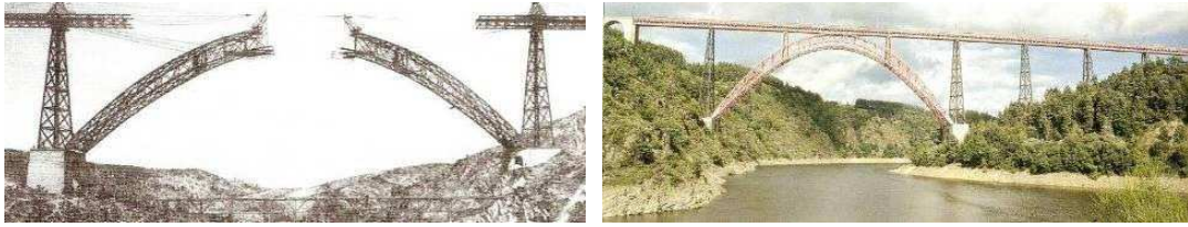
4. 41 Garabit Bridge, Gorge River, France, 166 m span, 1884, G. Eiffel
