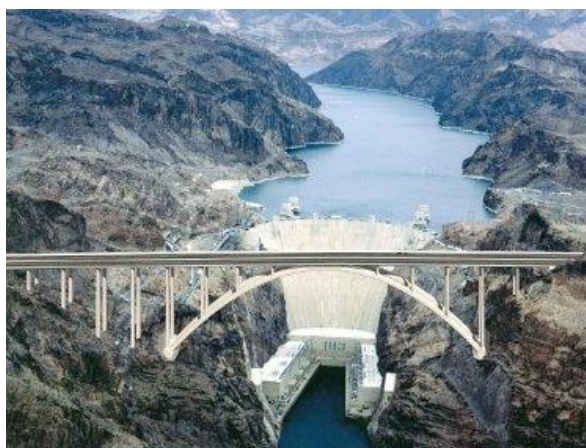
2. 36 Hoover Dam Bridge, Nevada, USA, 2004, 255 m span
