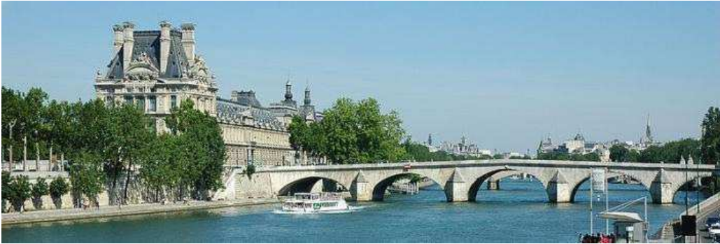
1. 29 Pont Royal, Paris, France, 20.58 m - 22.70 m - 23.52 m - 22.44 m - 20.64 m span, 1687, Jules Hardouin Mansart
