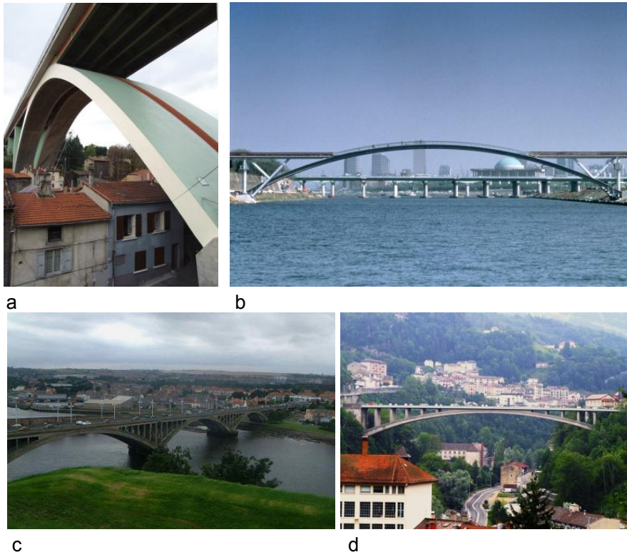
2. 39 a) Rive-de-Gier Bridge, France, 1964, 100 m span b) Seonyu, Seoul, South Korea, 2002, 120 m span c) Royal Tweed, Berwick-upon-Tweed, UK, 1928, 108 m span d) Saint-Claude Bridge, France, 1939, 130 m span
