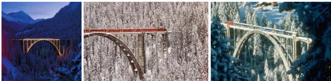
2. 6 Langwies Viaduct, Langwies , Switzerland, 1914, 100 m span, 42 m rise, K. Arnstein, E. Züblin
