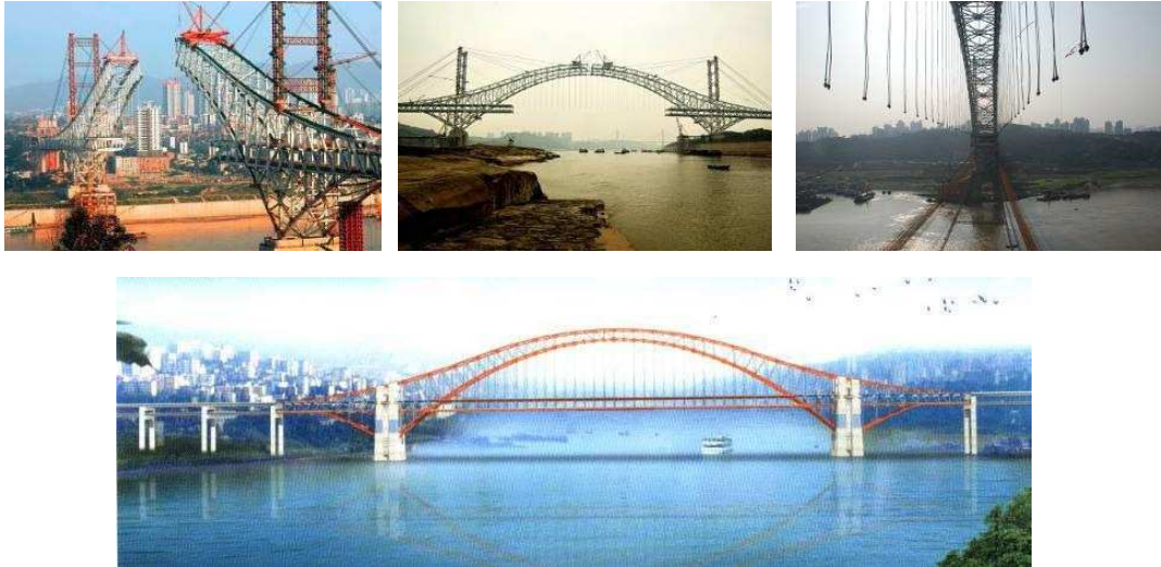
4. 39 Chaotianmen Bridge, located in Chongqing, 552 m
