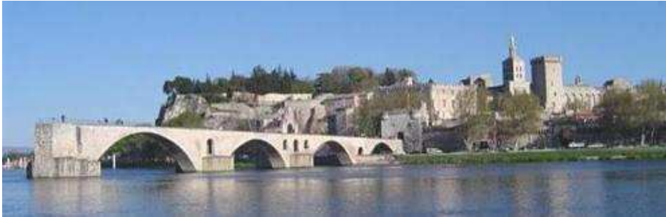
1. 19 Avignon Bridge, over the Rhone River, France, XVI century, 34 m span
