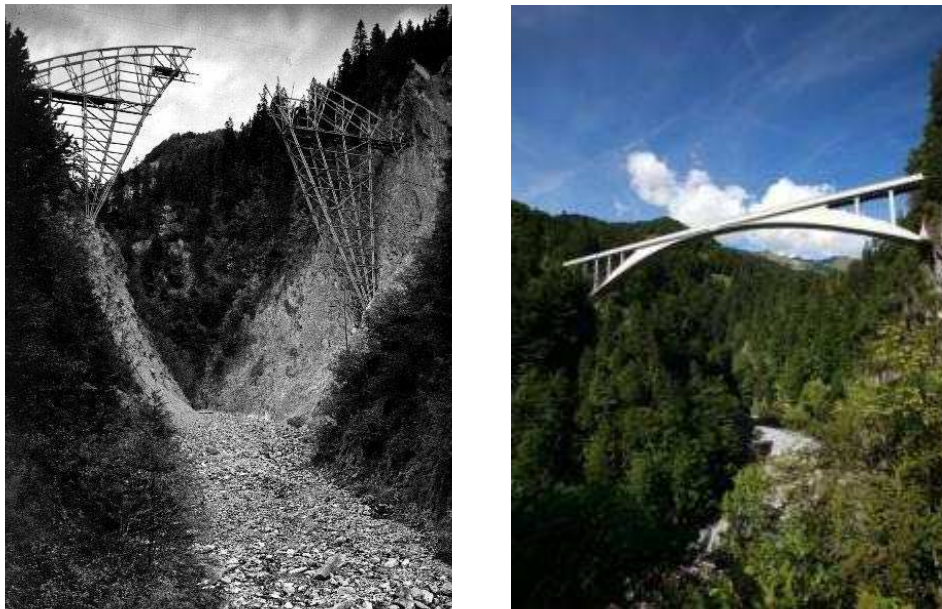
4. 10 Salginatobel bridge pictures: construction phase and state of art Salginatobel Bridge, Switzerland, 90 m span, 1930, R. Maillart
