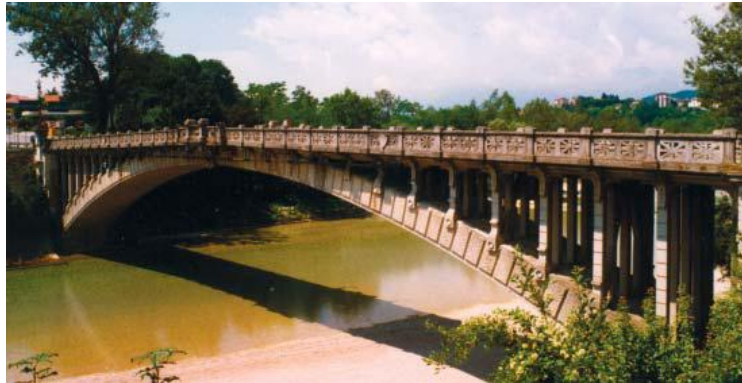
3. 46 Vittoria Bridge, Belluno, 1926, 72 m span, E. Miozzi
