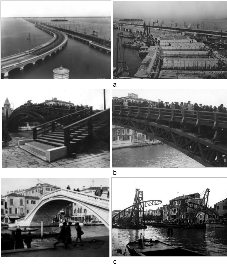
3. 45 a) Libertà Bridge, Venice, 1931-33, total length 4 km, E. Miozzi b) Accademia Bridge, Venice, 1932, 48 m span, E. Miozzi c) Scalzi Bridge, Venice, 1932-34, 40 m span, E. Miozzi
