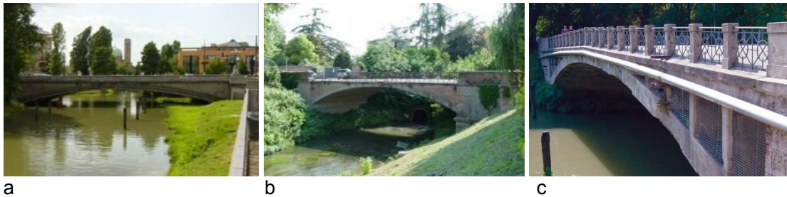
3. 42 a) Popolo Bridge, Padua, 1908, 43 m span, 4.35 m rise, A. Peretti b) S. Massimo Bridge, Padua, 1910, 15.5 m span, A. Peretti c) Ognissanti Bridge, Padua, 1921, 38 m span, A. Peretti
