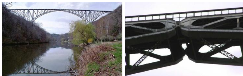
3. 15 Viaur Viaduct, 220 m span, 54 m rise, 1902, Carmaux, France, P. Bodin
