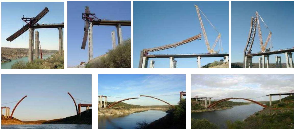
4. 64 Alconetar Viaduct, Spain, 2006, 220 m span, J.A.Llombart, J. Revoltós, S. Couto
