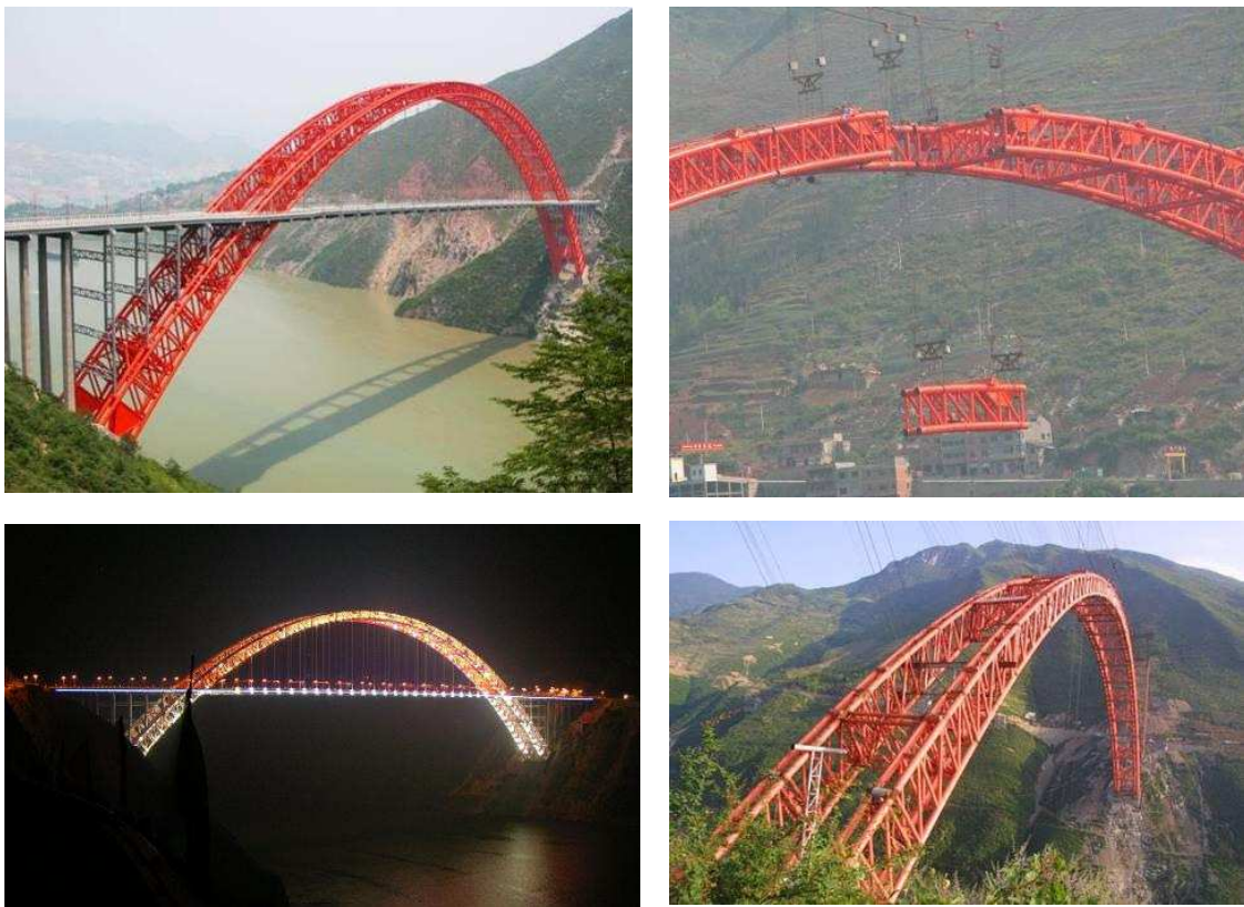
4. 48 Wuxia Yangtze River Bridge in Wushan, China, 460 m span, 2005
