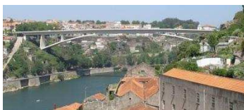
Infante D. Henrique Bridge Porto, Portugal 2002, 280 m span
