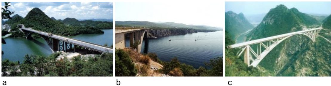
2. 37 a) Huayudong Bridge, Qingzhen, China, 1991, 150 m span b) Sibenik Bridge, Croatia, 1966, 246 m span, I. Stojadinovic, L. Gojkovic c) Jiangjiehe, Weng'an, Guizhou, China, 1993, 330 m span
