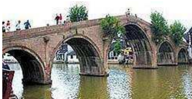
1. 11 Fengsheng Bridge, Zhu jia jiao, Shanghai Province
