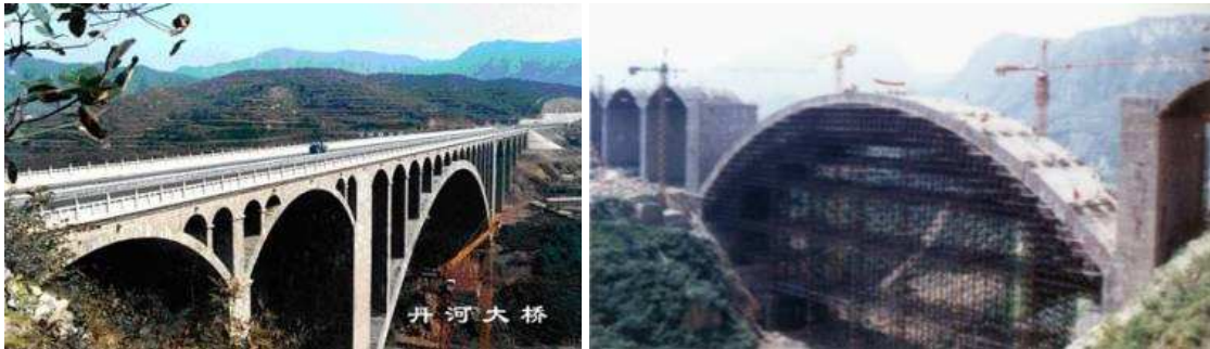
4. 6 Danhe bridge pictures: construction phase and state of art New Danhe Bridge, China, 146 m span, 2000
