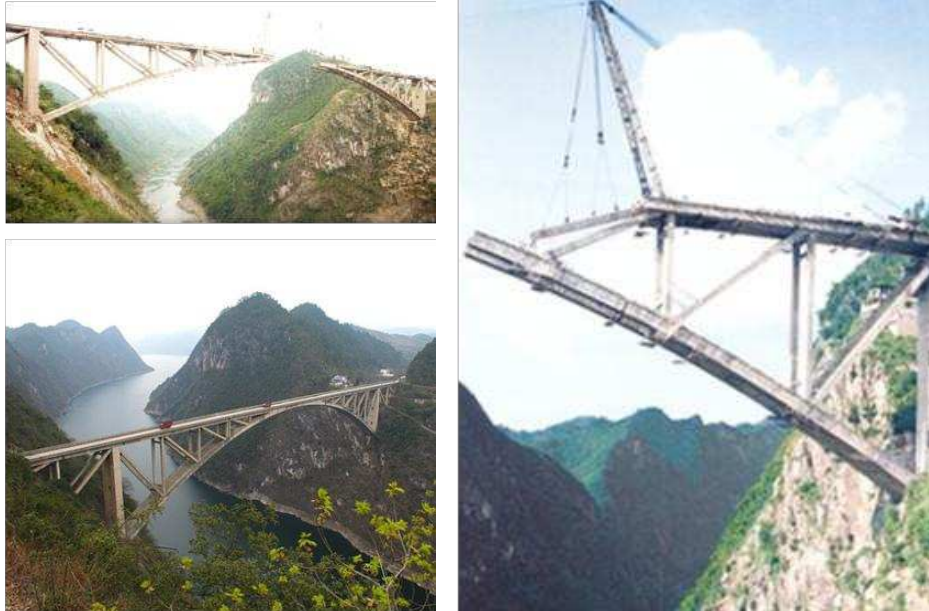
4. 37 Jangjiehe Bridge, Weng'an, China, 330 m span, 1995
