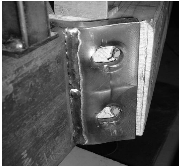
Fig. 12. Monotonic failure mode 2 observed in specimen P10 (without a glued-in steel plate): wood can produce prying forces in the end-plate
