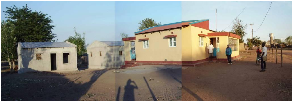
Figure 6.13. The old and the new housing compounds of household no. 4.
