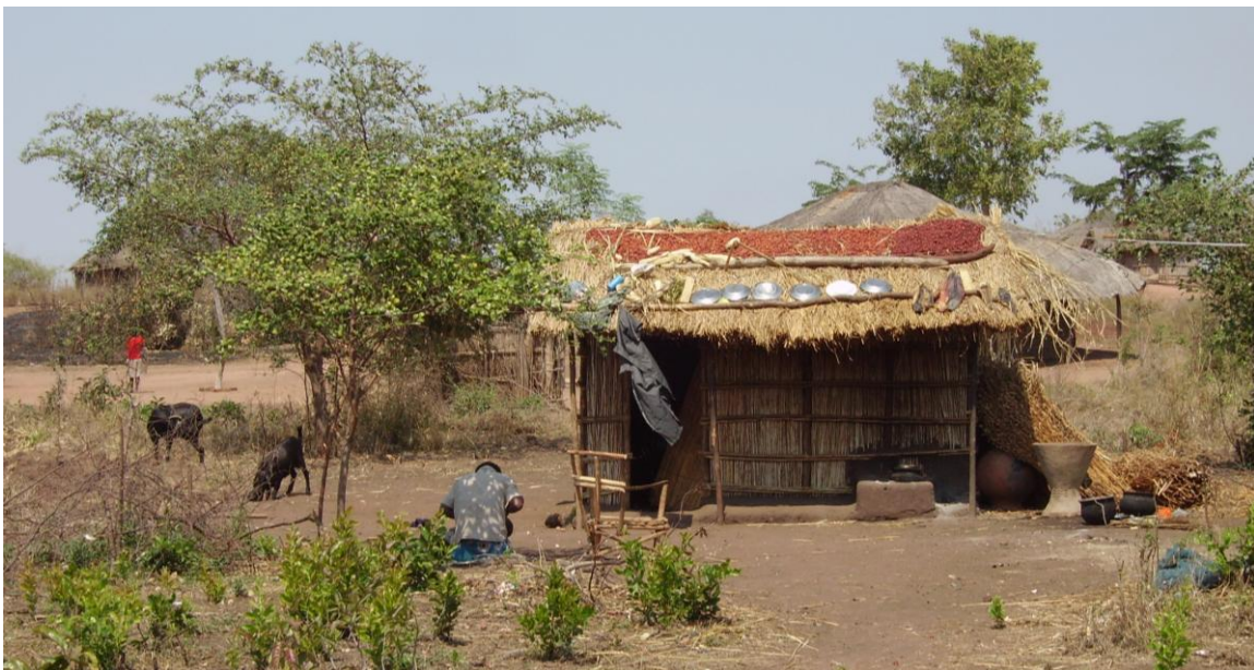
Figure 6.3. Palhota in caniço with straw roof
