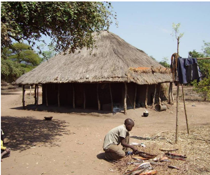
Figure 6.4. Palhota in adobe with a four-pitches straw roof and porches
