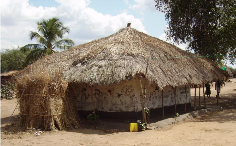
Figure 6.2. Palhota in adobe with a four-pitches straw roof
