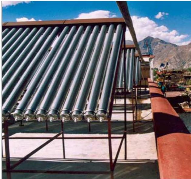
*Figure 1: Evacuated Tube Solar Collector in Tibet, China.*
