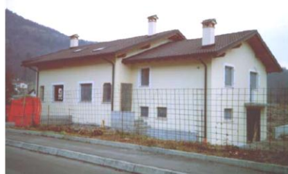
Fig. 2.7. One-family house in San Gregorio nelle Alpi (BL, Italy) (Mosele, 2009).
