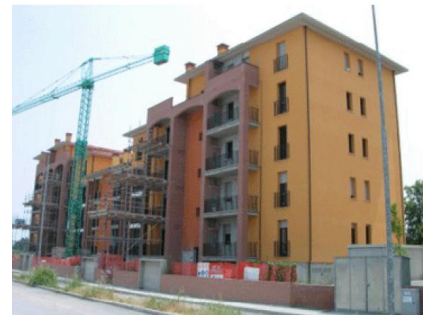
Fig. 2.8. Residential complex in Colle Aperto (MN, Italy) (Mosele, 2009).
