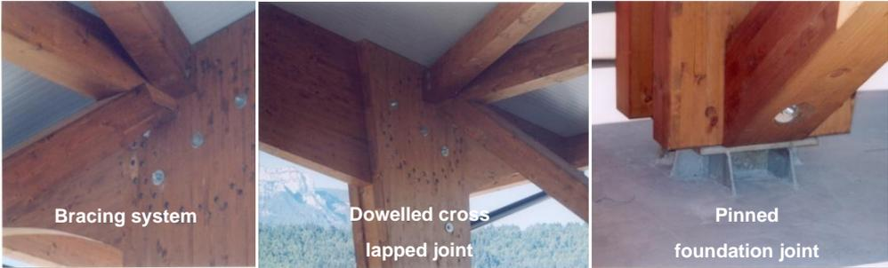
Figure 2.11 (a) Three-dimensional view of the Timber Portal frame system with dowelled cross-lapped joints (so-called “heavy timber structure”); (b) Details of an industrial warehouse built in Trentino (Italy)
