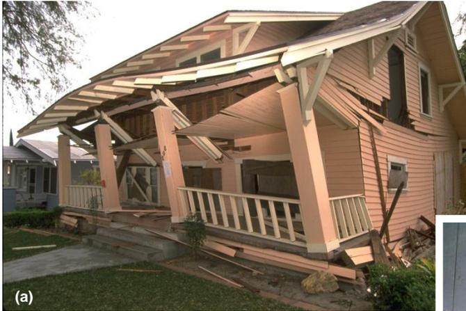
(a) and (b): damage to wooden buildings after the Northridge Earthquake; California, 1994 (FEMA 2010)
