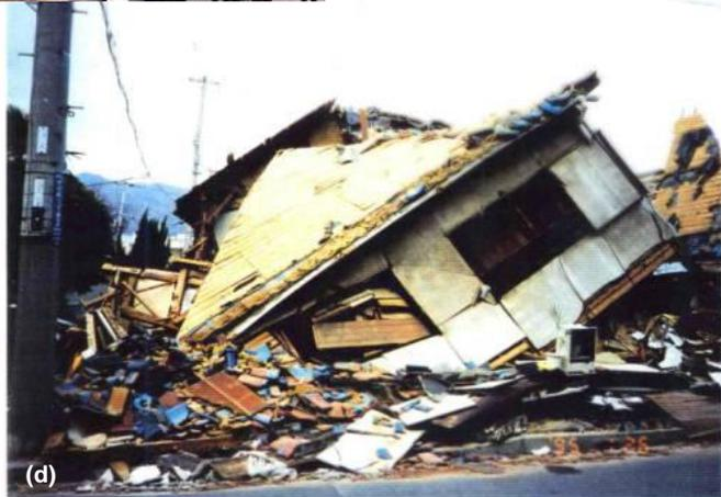
Figure 1.1. Overview of building damage after recent two earthquakes: Northridge 1994 with Magnitude of 6.7 and Kobe (Hanshin-Awaji) 1995 with Magnitude of 7.2 (Richter scale)
