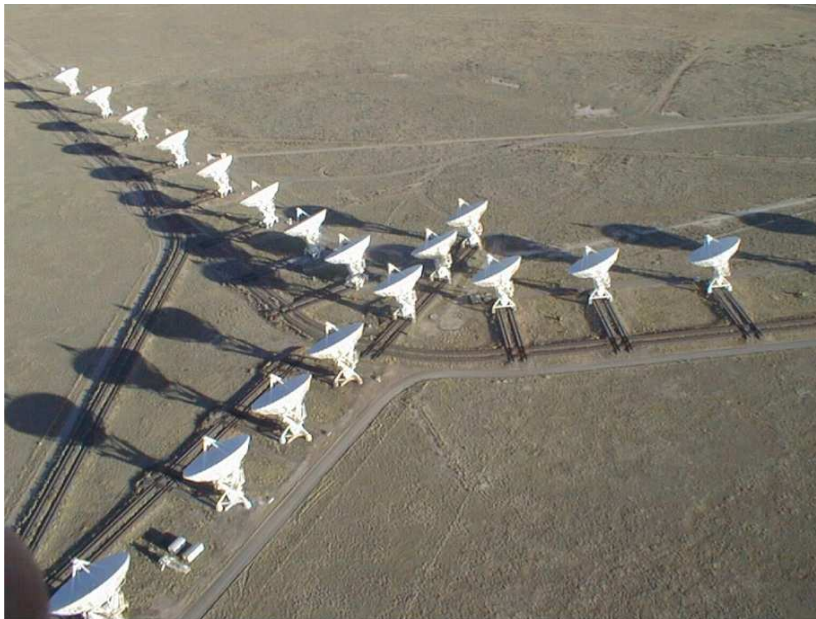
Figure 4. Introduction - The VLA, an array of 27 elements, each a 25-m paraboloid, is a Y-shaped array having three equiangular linear arms of 21 km.
