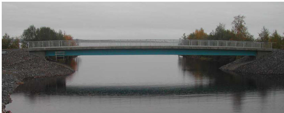
Fig. 15 Bridge over Leduån, Sweden – Composite Bridge with Single Span of 40 m (Nilsson, 2008)
