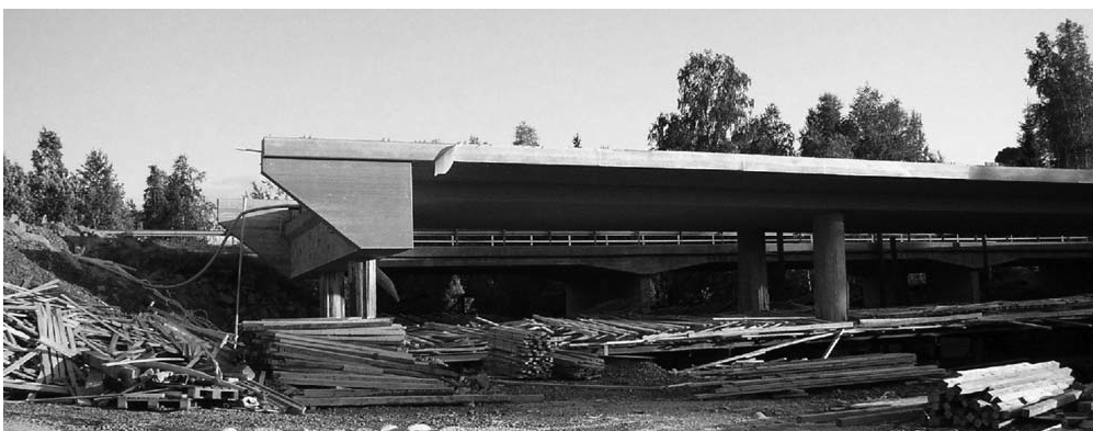
Fig. 116 Haavistonjoki Bridge, Finland, during Construction (Kerokoski & Laaksonen, 2005)
