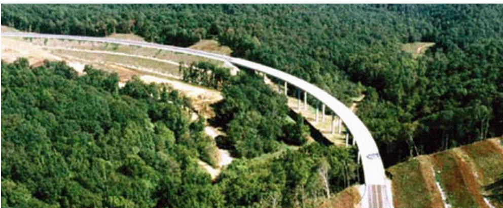
Fig. 8 State Route 50 over Happy Hollow Creek, Tennessee, USA
