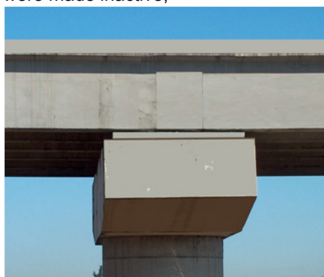
d) new slab was concreted.
