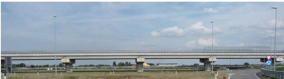
Fig. 50 Isola della Scala Bridge after Opening
