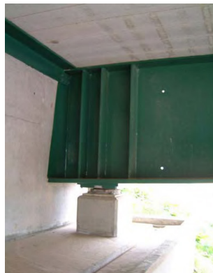
Fig. 11 Examples of Girder End Detail Used in UK (Iles, 2006)
