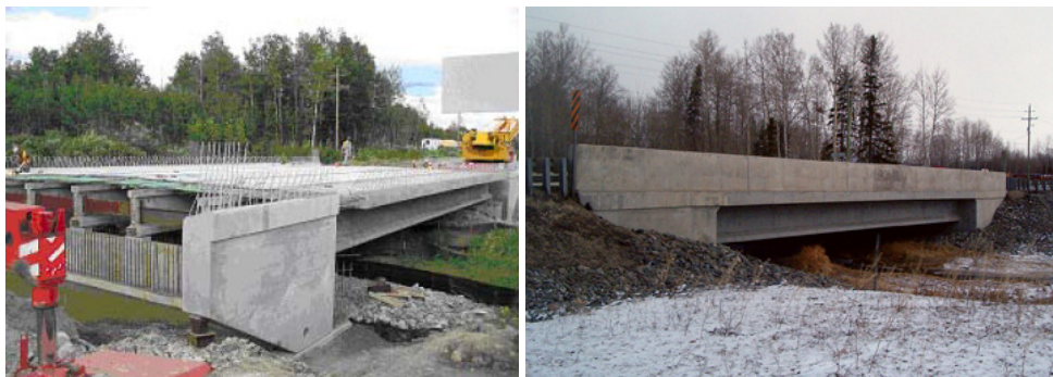
a) construction before cast-in-place concrete; b) as built
