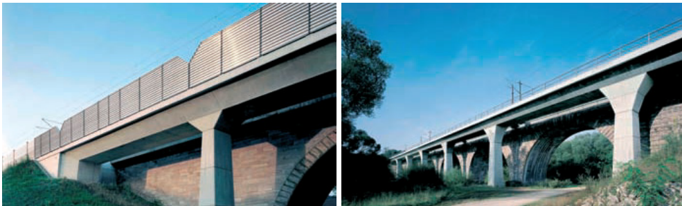
Fig. 17 Viaduct Rednitzal: Monolithically Connected Superstructure with Pier and Abutment (Marx & Seidl, 2011)
