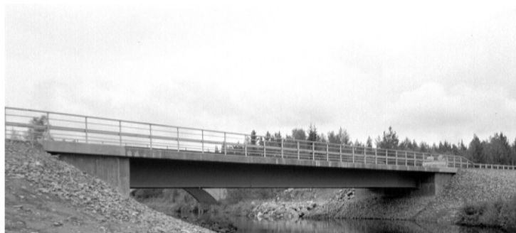
Fig. 14 Bridge over Fjällån, Sweden (Pétursson & Collin, 2002)
