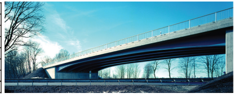
Fig. 16 Slenderness for Integral Abutment Bridges Used in Germany (Feldmann et al., 2010)
