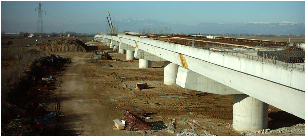
Fig. 49 Isola della Scala Bridge during Construction
