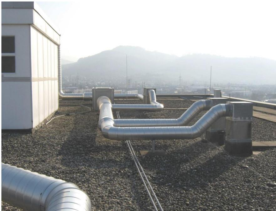
**Figure 5.4** Extractor chimneys and extractor fans on the flat roof
