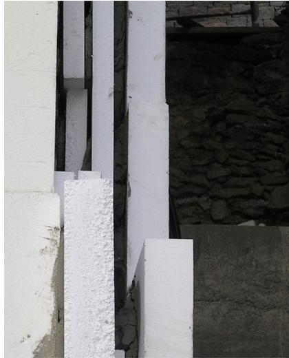
**Figure 4.4:** *Thickness variability of insulation layer in a building retrofit*
