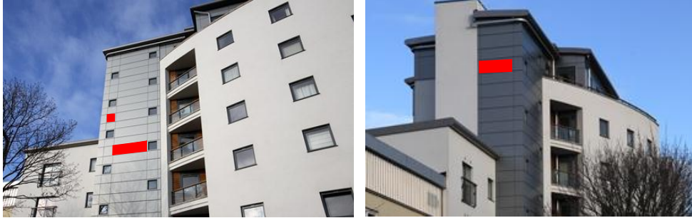
Figure 5.5: Residential building with cassette system, Cable street, London [Source: www.euroclad.ie/applications/residential.asp ]. Two cassette elements with different size are emphasized in red.
