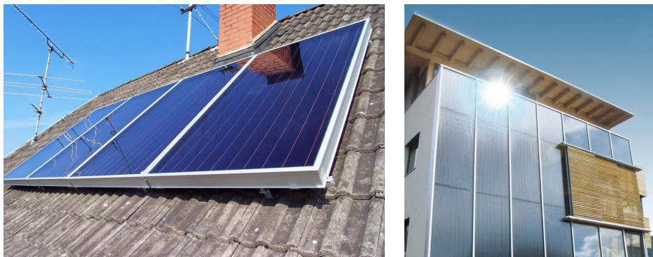
(a) Flat plate collectors installed on the roof
