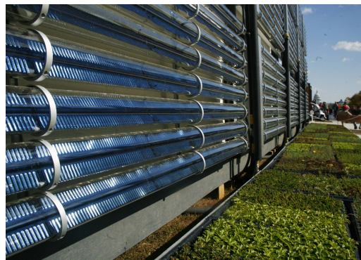
Figure 2.14: Solar Decathlon 2007, Cincinnati University, Evacuated tubes on the south facade of the team's house [credit: Kaye Evans/Solar Decathlon]
