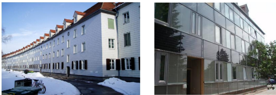
(a) Before the renovation of buildings (1959) - Graz (A) (b) After the renovation with installation of ST collector on the south oriented facade - Graz (A) [13]
