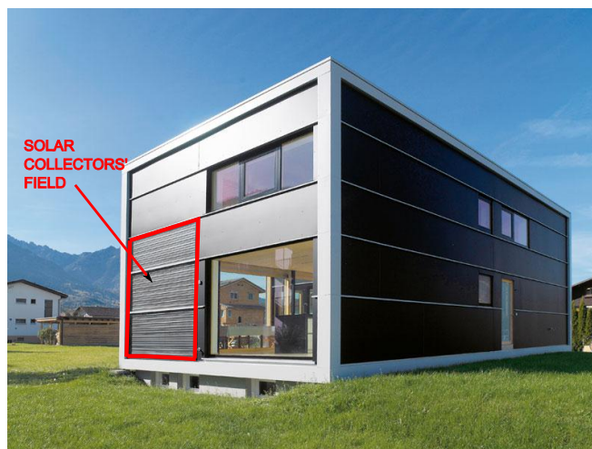
Figure 2.29: example of ST collectors integrated in facade, single family house, Nenzing (A), AKS Doma [credits: aksdoma.com]
