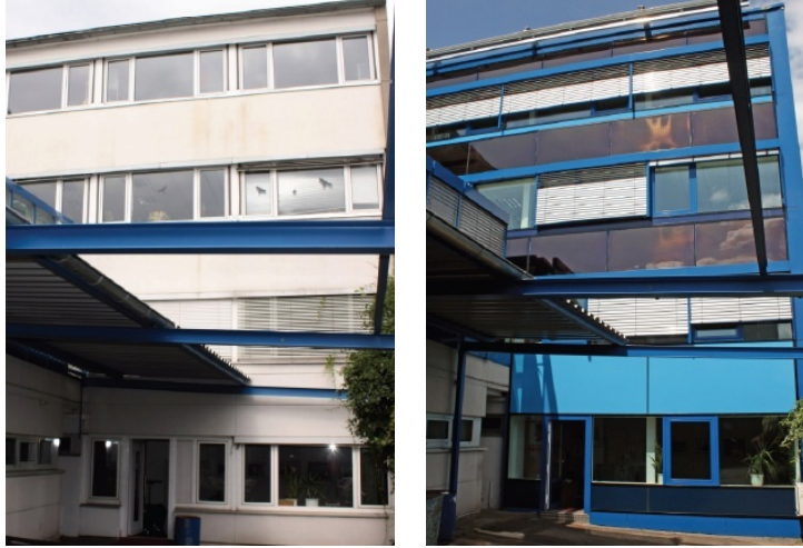
(a) South facade of the head quarter of Lamparter Stahlbau GmbH & Co. KG before the renovation in 2008. (b) The building after the renovation.
