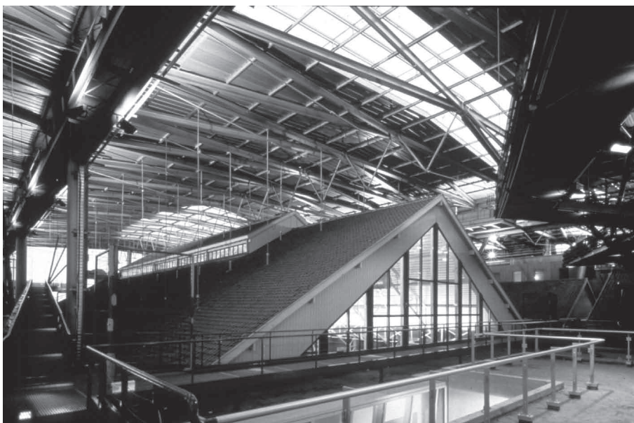
B. Tschumi, Contemporary arts center "Le Fresnoy", Tourcoing (France, 1987).
