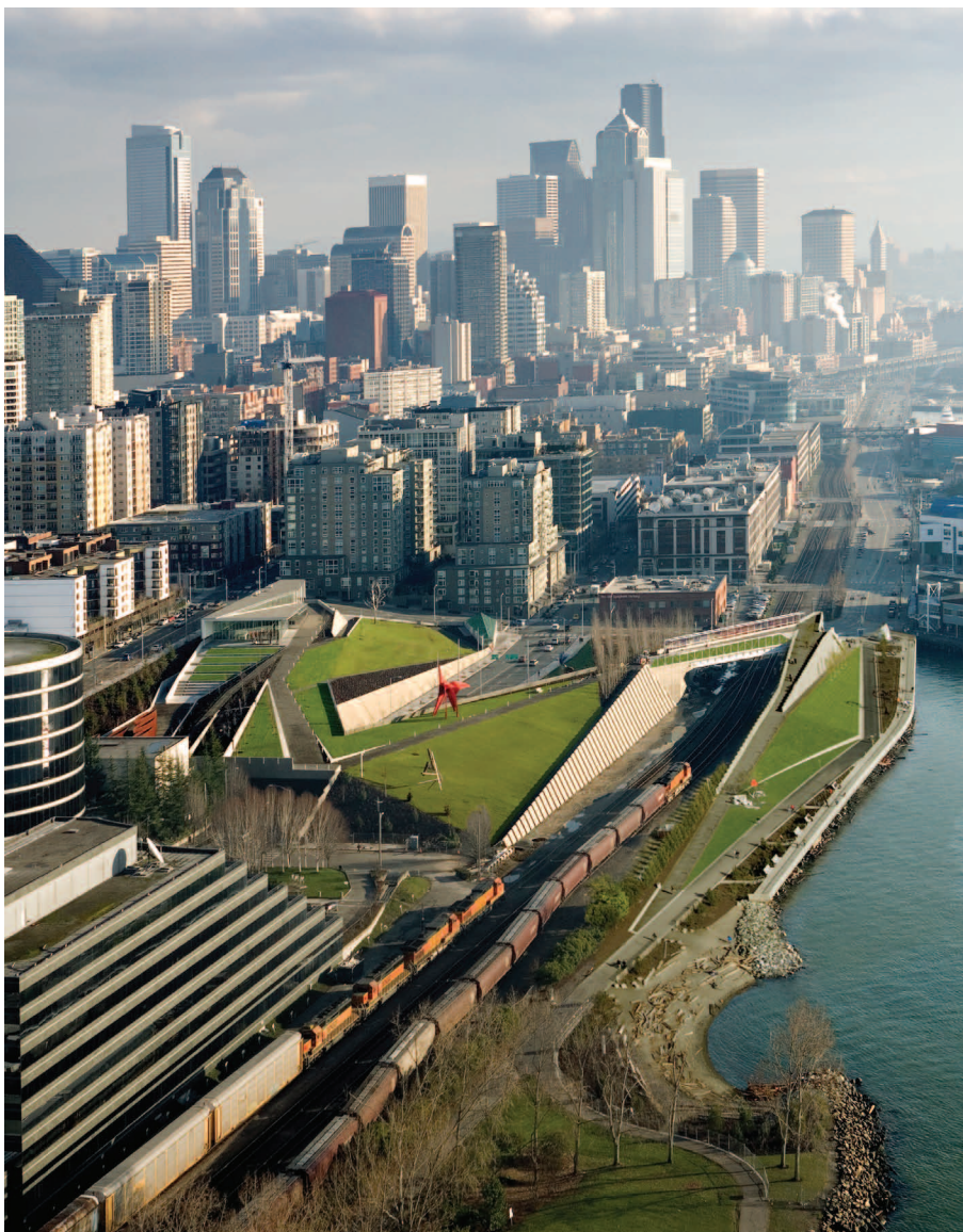
L. Halprin, Freeway Park, Seattle (USA, 1976). Perspectives recall from time to time the next frame.
