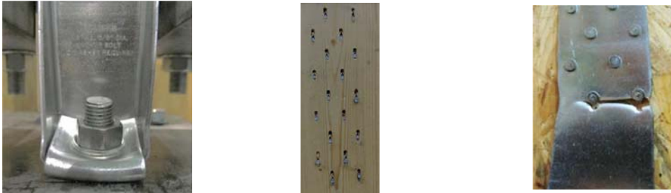
Figure 12 - Steel base deformation, nailed connection deformation and deformation of the vertical flange
