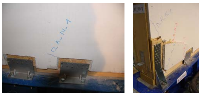
Figure 24: Some damages observed in the test S_ST_RIV1
