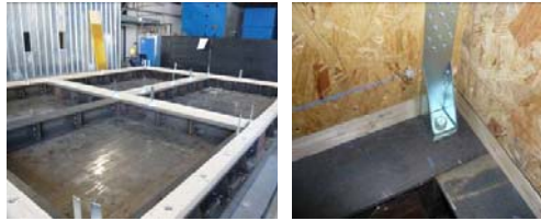
Figure 9: Grid of steel beams arranged in correspondence of the structural walls
