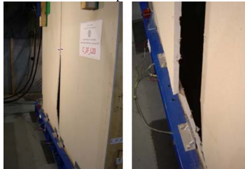
Figure 15: Out of plane failure of the GFB panel
