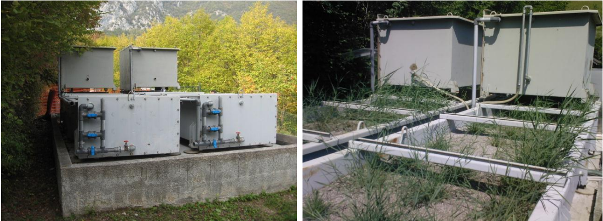
Figure 28 View of the pilot Plant in March 2010.
