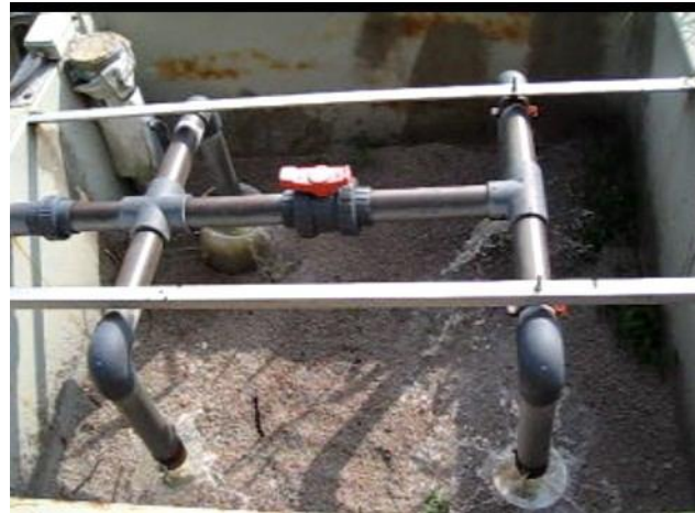
Figure 23 Distribution system above the VSSF on both lines: E-line and C-line.
