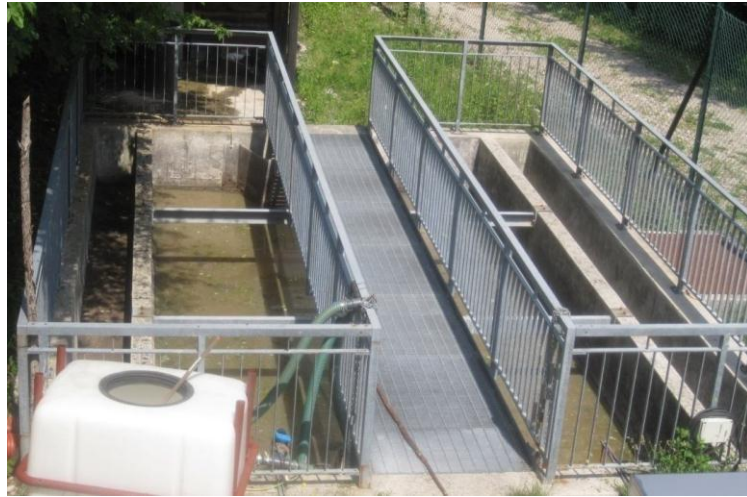
Figure 21 View of the Imhoff tank
