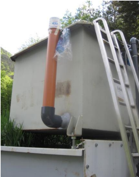
Figure 27 Piezometer pipe where the level probes are installed in the E-line
