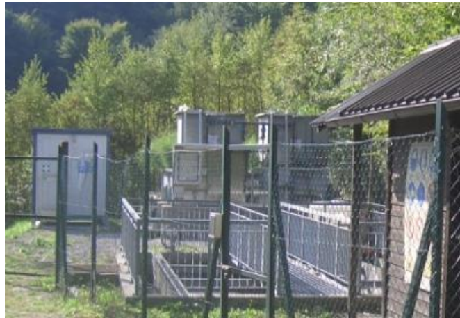
Figure 20 View of the pilot plant installation
